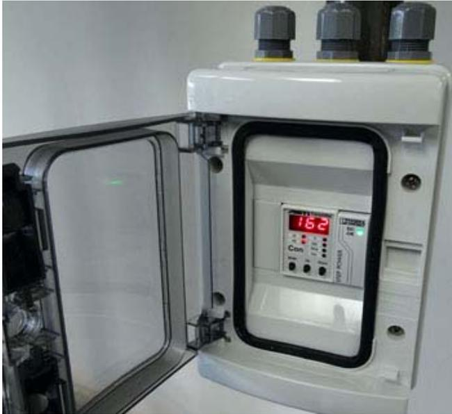
**Single Channel Contacting Conductivity Transmitter**
